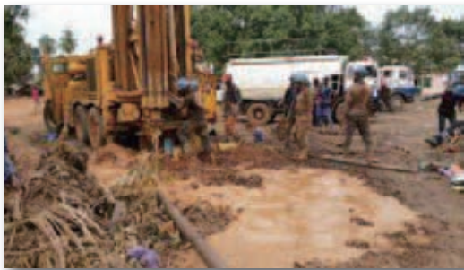
Well drilling project at Bokai District
