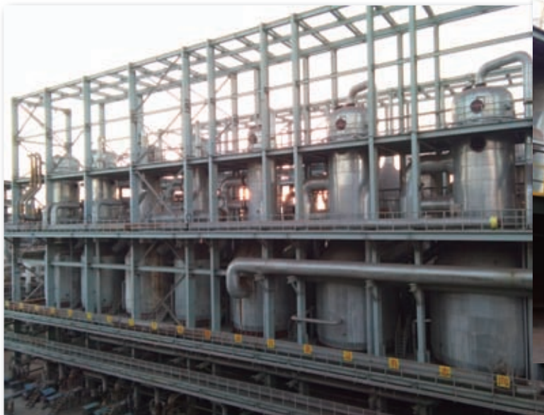
Conversion of six-effect evaporator to seven-effect evaporator
